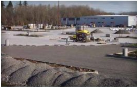
Figure 1. Mechanical installation speeds PICP installation.
