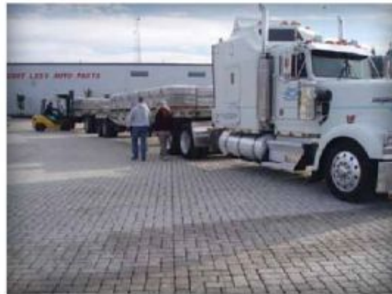
Figure 4. PICP can withstand heavy truck loads. Since PICP requires no curing, this truck delivered pavers on a completed area of PICP to support construction of the remaining area.
