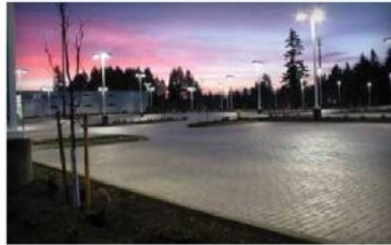
Figure 2. The completed project was submitted for LEED® silver certification. The paver's solar reflective index of 39 and the PICP's ability to reduce runoff and pollutants contributed to LEED® credits.
